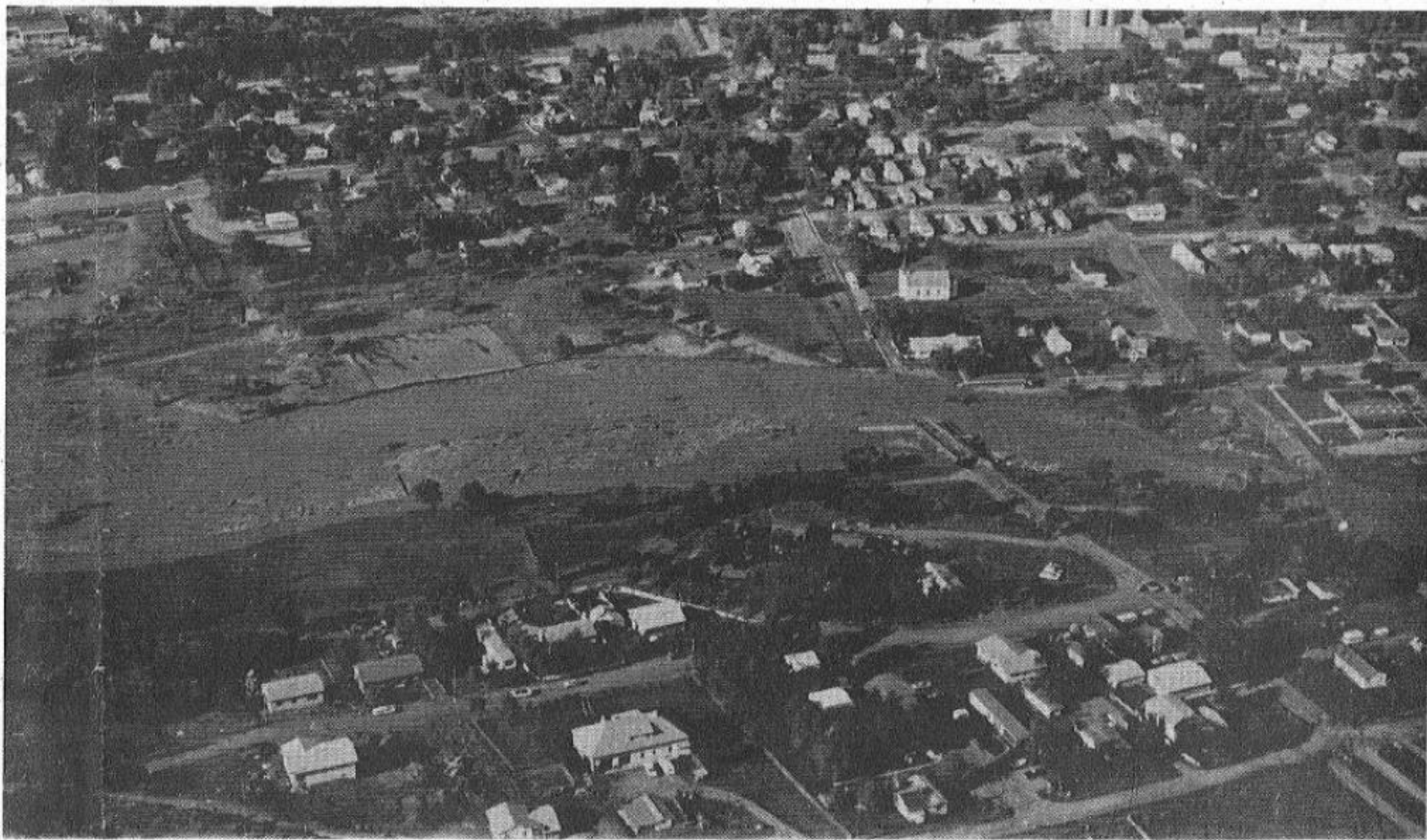
This aerial view by Gary Coe shows Bear Butte Creek where it carried away the Seventh Street bridge approach and part of the new tennis court erected in the floodway.
